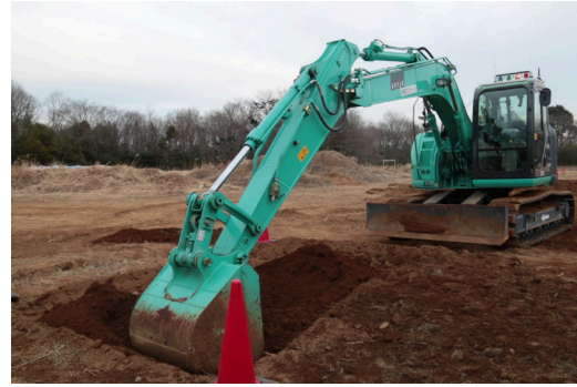
Figure 9: Digging the land and filling
